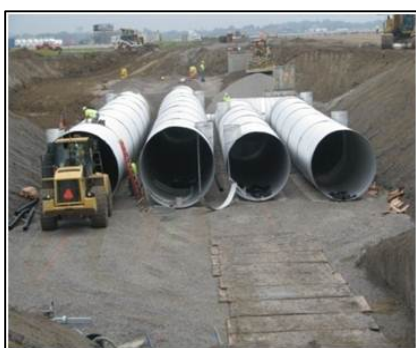
Underground Stormwater Management Facility Under Construction
