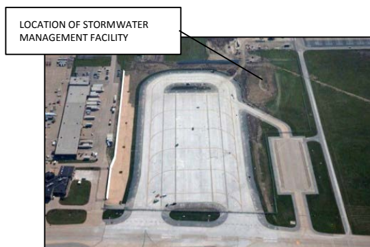
Taxiway Q and Hold Pad
