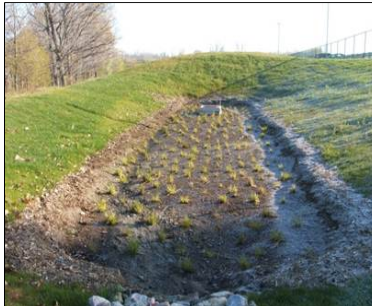
Riveredge Bioretention Cell
