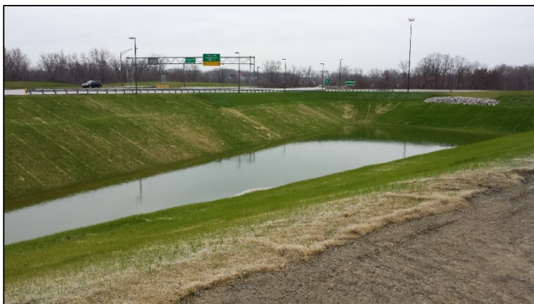
South Retention Basin (Photograph Taken 11/21/2013)
