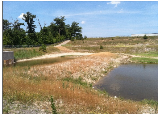
North Detention Basin after 2012 Retrofit
