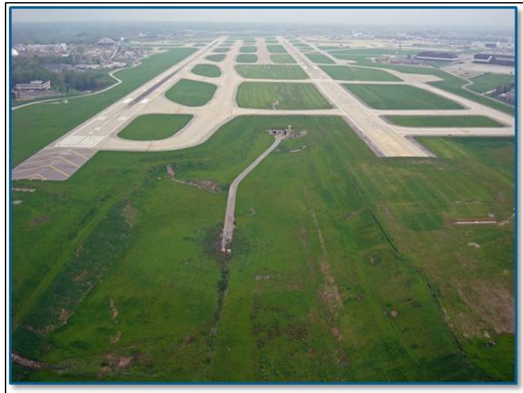
Central Detention Basin
